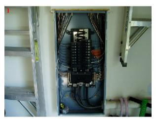
Main / Service Disconnect Location - Main Disconnect Located at Main Service Panel
