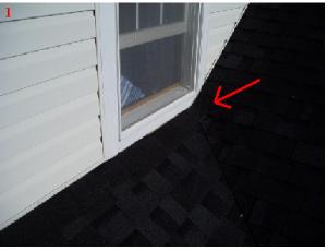
Flashing Type - Aluminum, Galvanized, Plastic / Neoprene
